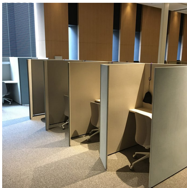
Installation of individual booths
