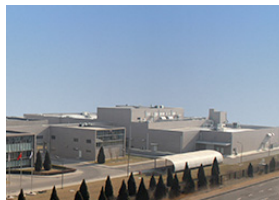
Pharmaceutical production building, Tianjin Tanabe Seiyaku
